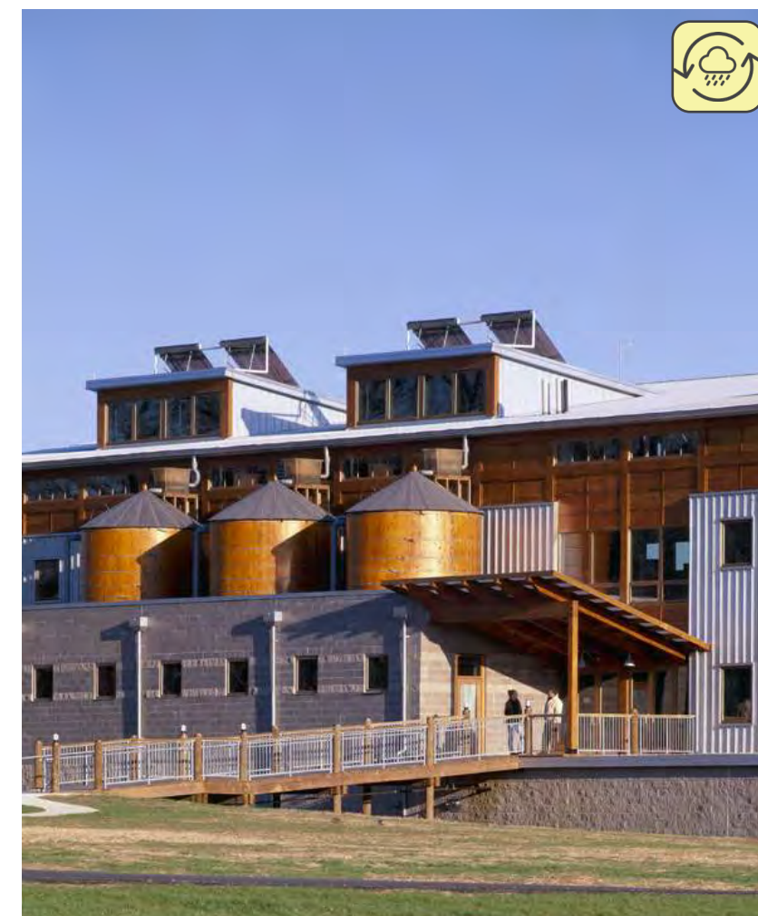
4. Rainwater Collection Cisterns | CBF Philip Merrill Environmental Center
