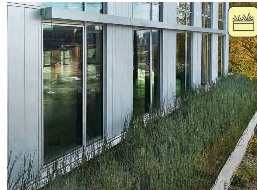
5. Constructed Wetlands | Bullitt Center (Credit: The Miller Hull Partnership)
