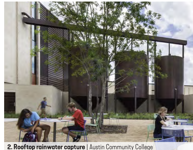
2. Rooftop rainwater capture | Austin Community College
